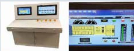
Power house control Console, remote access screen & monitor panel displaying all five generators in sync.
